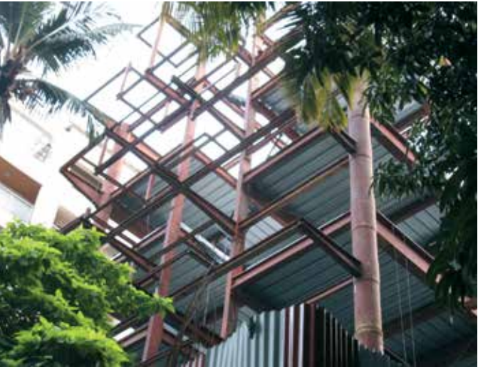
This page above: the building during construction phase – fabricated steel columns and beams were brought into the site in sections and raised quickly. Left and below: the greys on the building facade give way to fresh and lively interior surfaces (as seen in the last spread)
